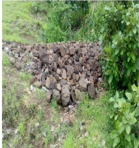
after work done
