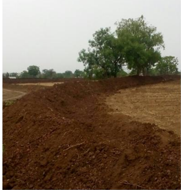
after work done
