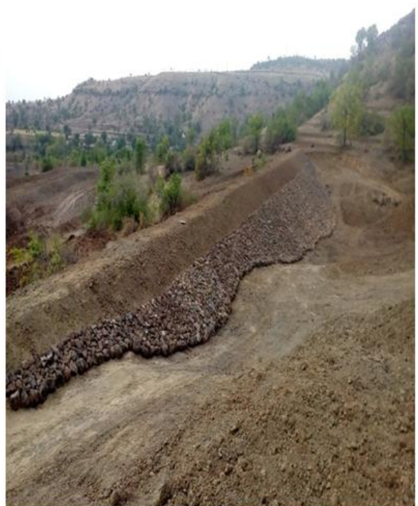
after work done
