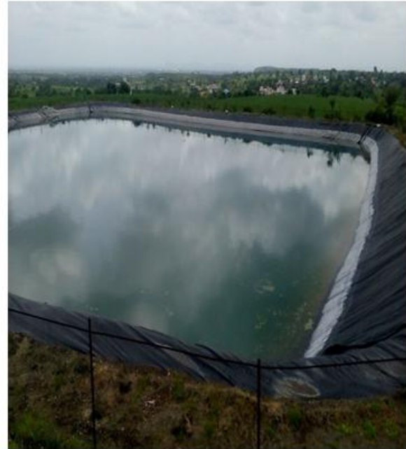
after work done
