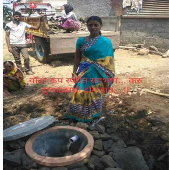
after work done
