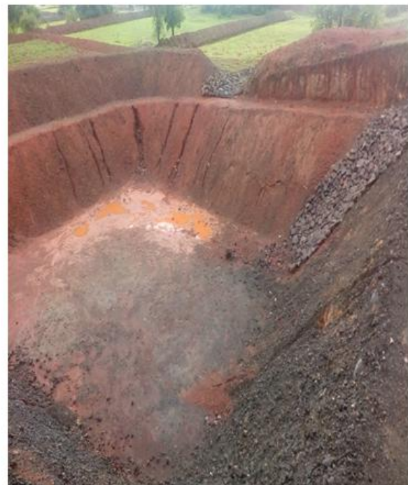
after work done
